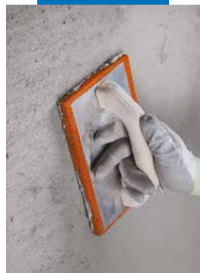
2Pressun á Planitop Smooth & Repair
